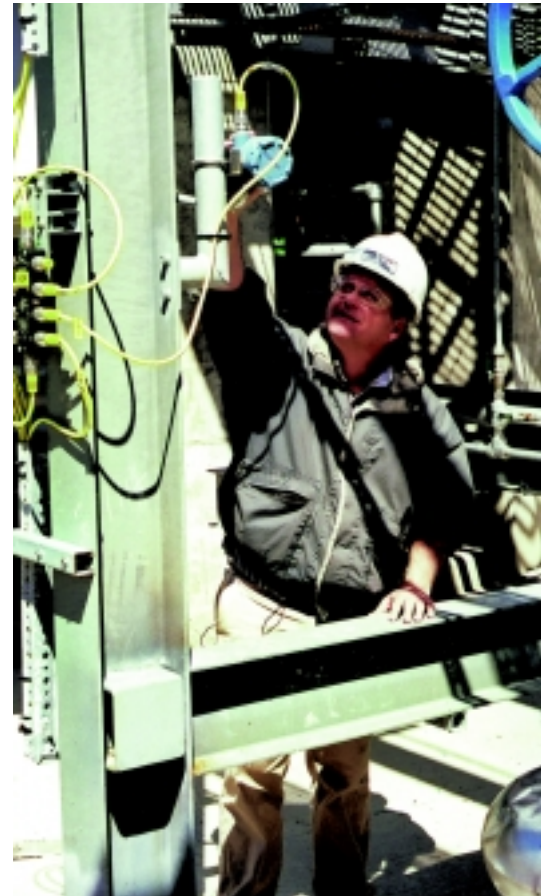
A well planned maintenance strategy can minimise costly equipment downtime.
